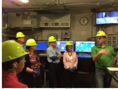
Cargill plant manager Ryan Fifield explains the plant operating systems to legislative tour participants. State Senator Tony Avella of Queens (center) was one of the attendees.
